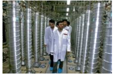
Stuxnet Iran nuclear plant
