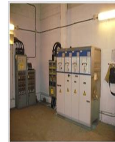
Secondary Substations with Telecontrol
